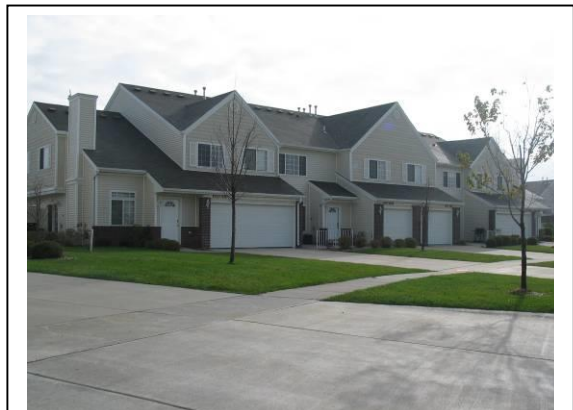
Example of Single-Family Attached
